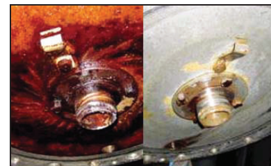
Vessel cover contaminated
